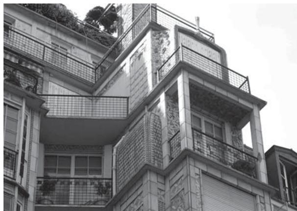
Figura 21 - Terraços e lajes em balanço. (Fonte <[http://bp2.blogger.com/\\_J5I22IvGFu8/RloEQPLKBSI/AAAAAAAAAko/gzP3K4p0abI/s1600-h/IMG\\_1024.jpg](http://bp2.blogger.com/_J5I22IvGFu8/RloEQPLKBSI/AAAAAAAAAko/gzP3K4p0abI/s1600-h/IMG_1024.jpg)> Acesso em 21 de setembro de 2007).
